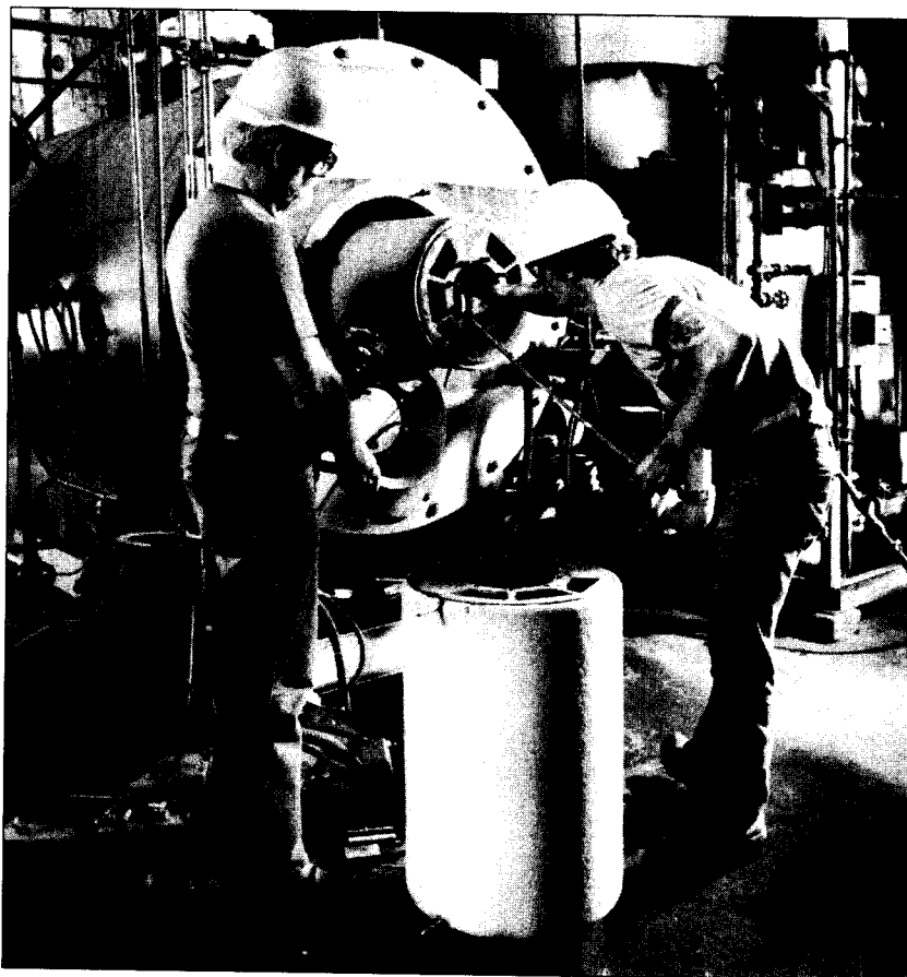
Figure 15.17 Ceramic fiber burner being installed in high-pressure steam boiler. | SOURCE: Courtesy of the Gas Research Institute.
